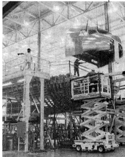
Test version of 777 nose section confirms that team-oriented, computer-design processes work. The section is being built as final verification that parts designed and 'preassembled' electronically fit the way they do on the computer screen.
